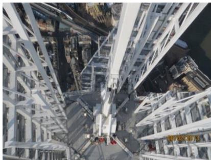
View from the top during installation
